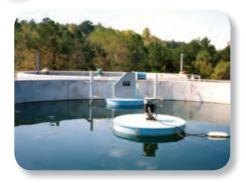
Flow enters the bioreactor where a series of independent phases promote biological treatment. Separate mixing and aeration devices allow the contents of the reactor to undergo biomass conditioning and nutrient reduction by alternating aerobic and anoxic periods. Following settling, supernatant is transferred from this first barrier to the cloth media filter.
