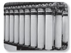
Flow enters the membrane modules where low positive pressure enables the fluid to permeate the membranes, excluding fine particulates. Filtrate is directed to final discharge or a reuse application.
