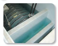
Flow enters the cloth media filter where TSS, turbidity, and particulate (insoluble) phosphorus are reduced to very low levels, achieving a high-quality effluent that can be used in many reuse applications. The filtered water is transferred from this second barrier to the ultrafiltration membranes.
